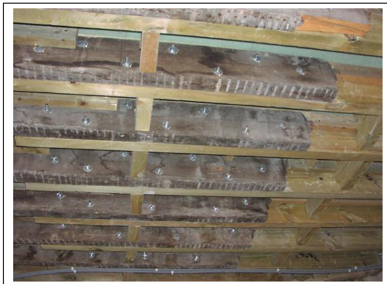
Strengthening of existing floor joists at 36&38 Tavistock Street
